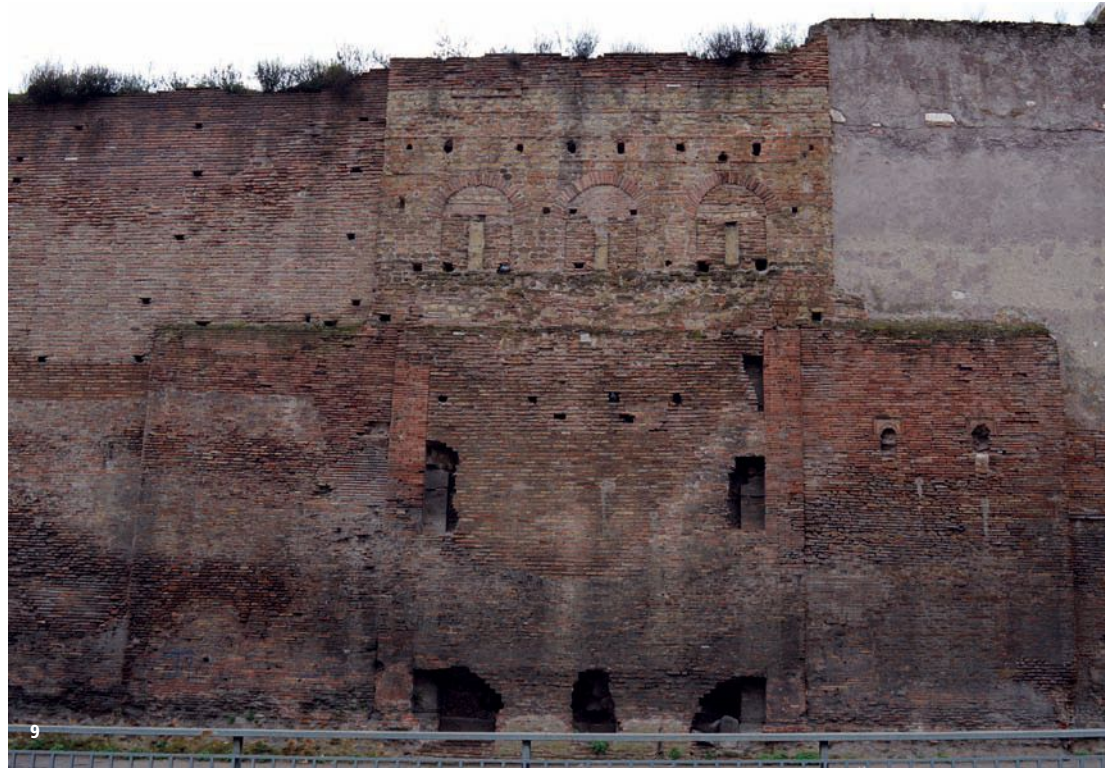
9. The remains of the Castra Praetoria's single portalled north gate, Porta Principalis Dextra (probably filled in by Maxentius). The lower walls are Tiberian, the upper walls date from circa AD 270–75 and the tower from circa AD 238.
